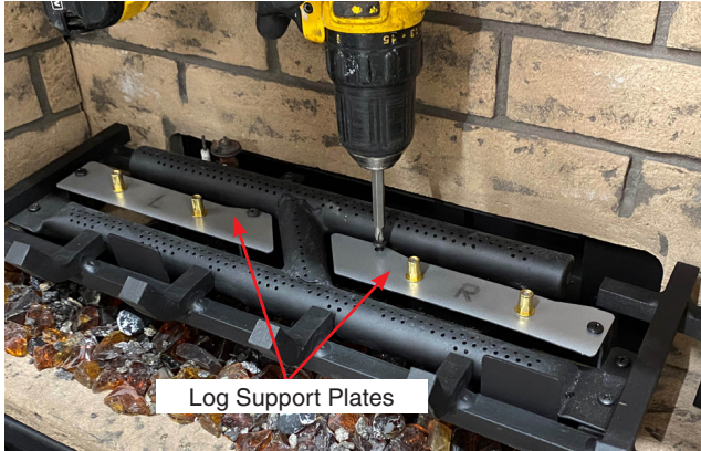
Diagram 5-Install Log support plate installation
