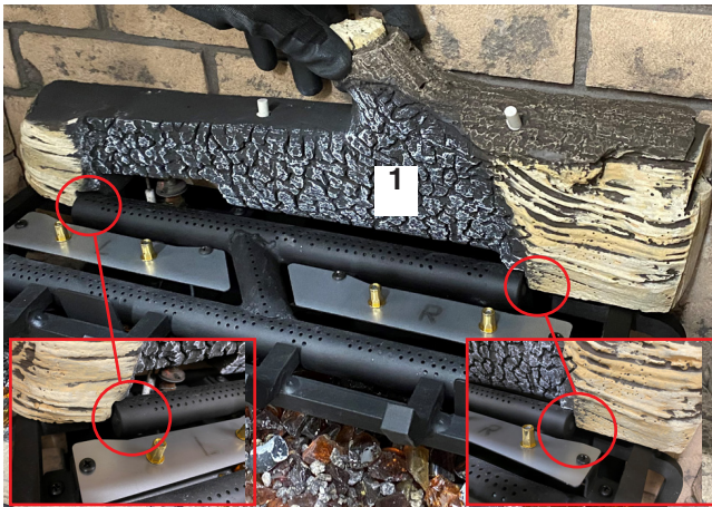
Diagram 6-Log 1 installation
