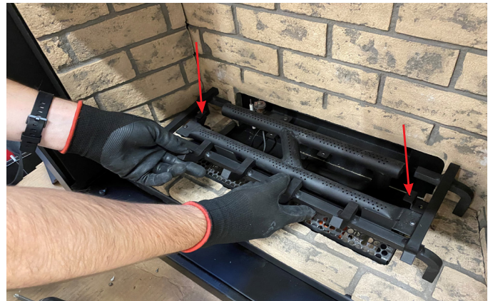
Diagram 2-Log Grate Install
